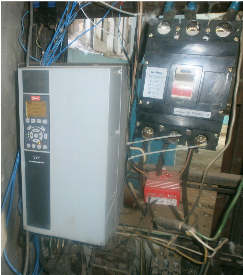
Figure 1 – General view of mounting the frequency converter and current transformer
